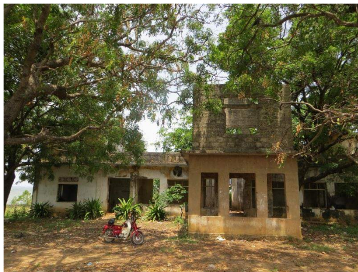
Photo 14: The proposed building to be renovated as a library by the diaspora
