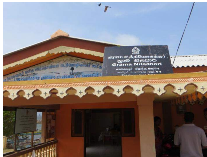
Photo 15: Village Community Center
